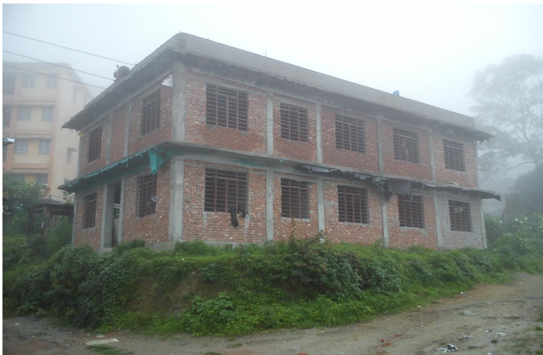
Newly Constructed Veterinary Hospital Bldg under ARD Deptt, at Kurseong
